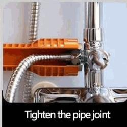
Tighten the pipe joint
