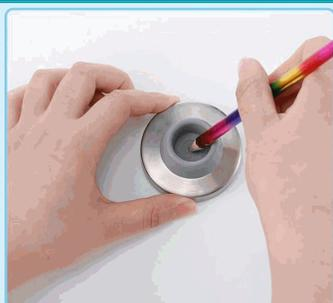
Step 1: Placed bumper assembly on wall so the door handle hits. Mark position of screw with a pencil through the center.
