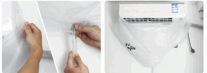
4. The sticker on the outside of the air conditioner is attached to the water receiving bag and inserted into the water receiving pipe.
