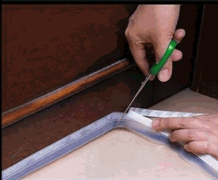
Cut into the proper length
